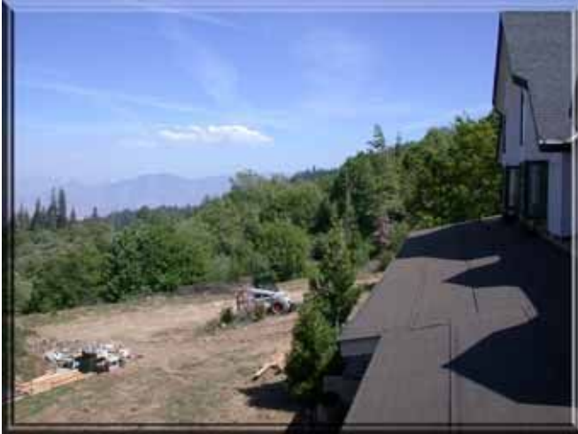
Figure 86: The rear of 8301 shows the stucco siding and just as important, the large area of defensible space on the downslope side of the house. A new composite roof was being placed on the house during the site visit. Notice the lack of tall conifers on this side of the house. This house is within the perimeter of the Alta Fire of 1973.
