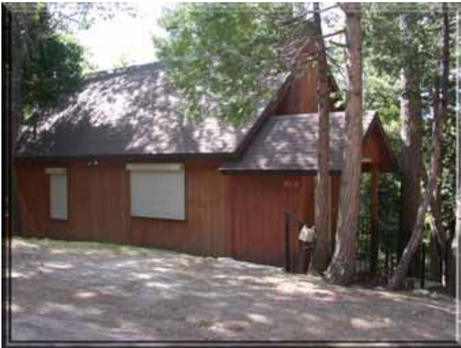
Figure 85: Metal shutters found on this cabin will provide wildfire protection to one of the more vulnerable components of the structure.
