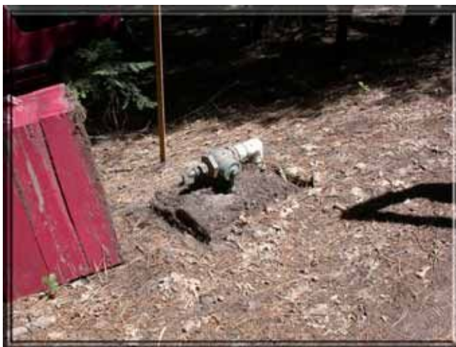
Figure 32: This is an example of what may be found under the red boxes. Fittings were not standard. In some cases, hydrants were buried under forest debris.
