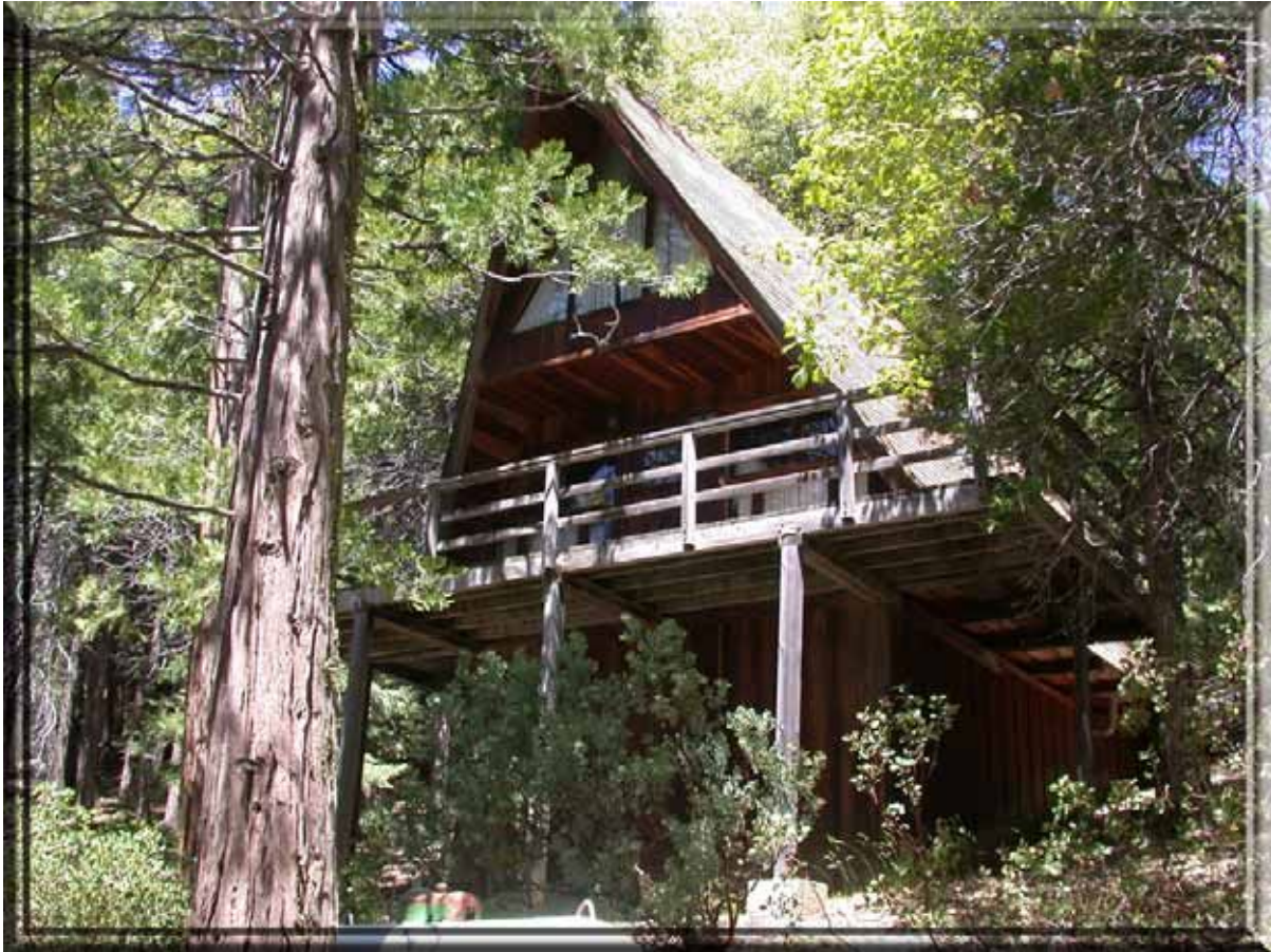
Figure 20: This home on Alta Sierra Road has a very hazardous deck with highly combustibile Manzanita in close proximity. A wildfire would cause burning material to either land on the deck or ignite it from below. Once the deck is aflame, the home will be jeopardized. Photograph by Timothy Walsh
