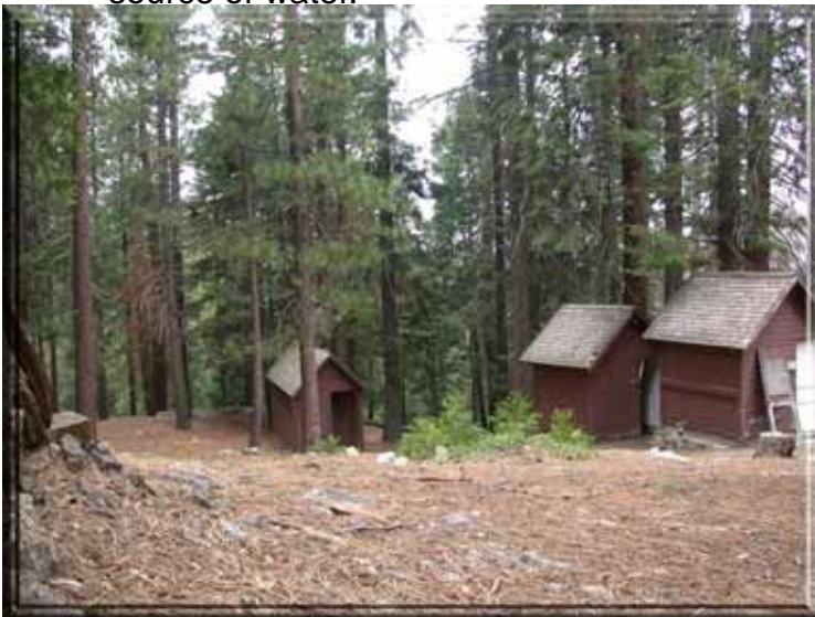
Figure 50: An example of some of the buildings at Camp Kaweah. They pose a hazard because they are covered with wood shingles (some have fallen off), doors are open or missing, and there is a heavy needle layer on the forest floor. Photo by Timothy Walsh.
