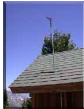
Figure 89: Sprinklers protect the pump house roof.
