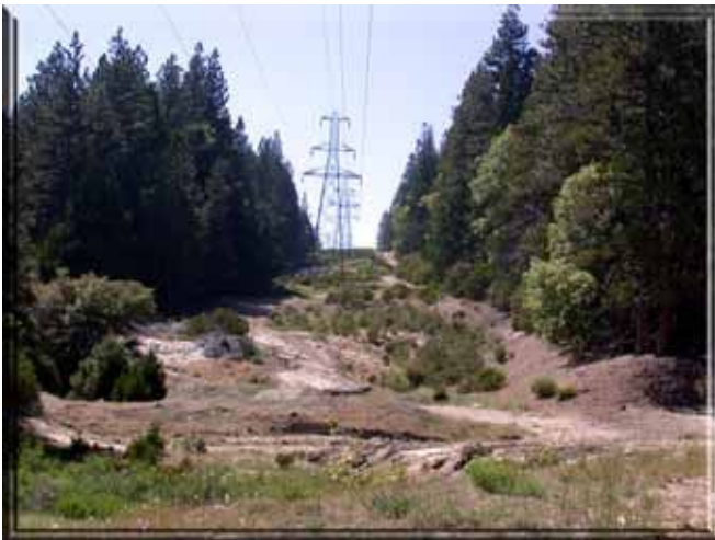
Figure 33: The fuel modification under the high-tension powerlines ranges between 60-80 feet wide. Photo by Timothy Walsh.
