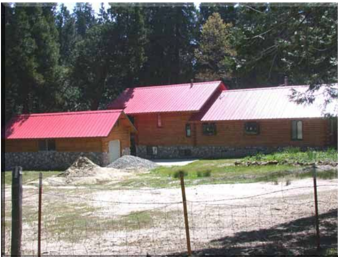
Figure 39: The structure located at 10880 Oak Way offers a large area of defensible space and no slope. One safety concern is the large tree leaning over the house and garage! Photo by Timothy Walsh.
