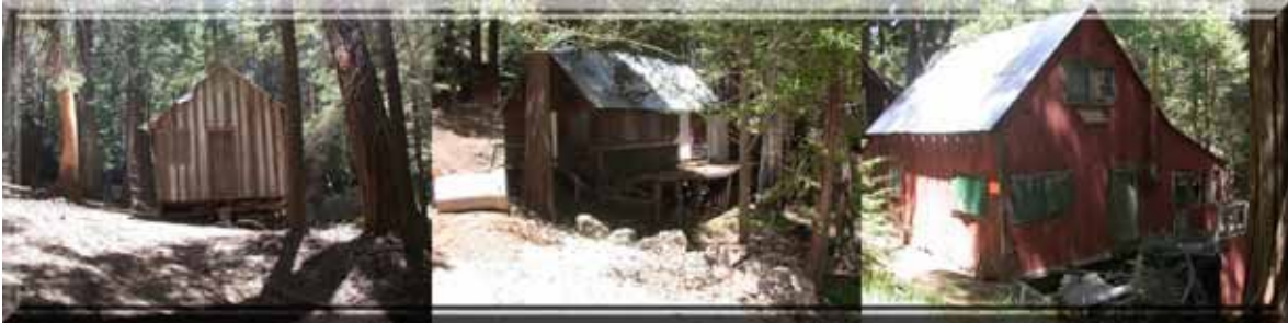
Figure 40: Small cabins that are condemned or should be will pose a risk to all of the structures around them. Photo by Timothy Walsh.
