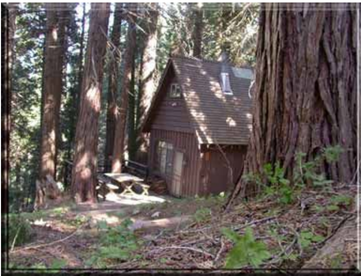
Figure 57: This is a typical cabin found in the Shirley Meadows Tract. Wood construction with a comp roof is the normal construction type. The area has very large trees with a large amount of duff and needle litter.
