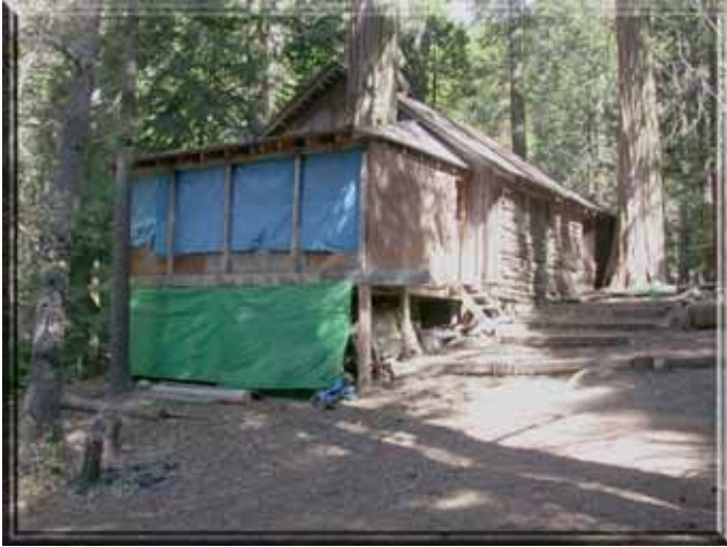
Figure 44: 2043 Alta Sierra Road is susceptible to ignition with plastic tarps covering plywood and wood stored under the covered porch. Photo by Timothy Walsh.
