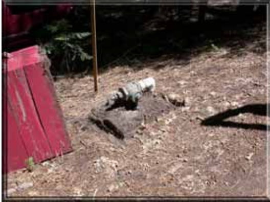
Figure 91: A “hydrant” that has years of forest debris underneath it makes operation difficult
