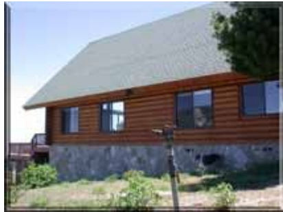
Figure 88: The house is made of logs with a rock fascia. The eaves of the home have been boxed in not allowing embers to be blown under them compromising the structure.
