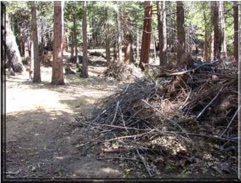
Figure 34: This photo is behind 1686 Locus showing slash piles and the excellent defensible space behind the structures. Trees have been thinned and the ladder fuels were removed. There is a good turnaround behind 1674 Locus. Photo by Timothy Walsh.
