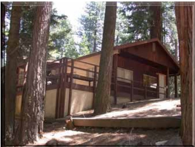
Figure 87: The deck at 308 Pine Drive has been completely enclosed using a fire resistant stucco covering.
