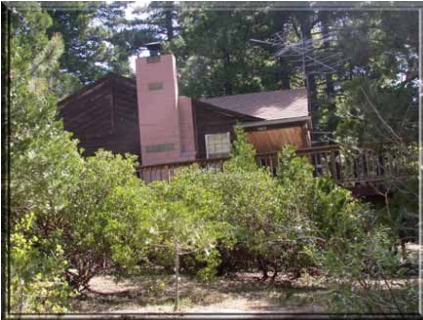
Figure 11: This house located on Ponderosa Drive uses highly flammable Manzanita for ornamental vegetation. Photograph by Timothy Walsh.
