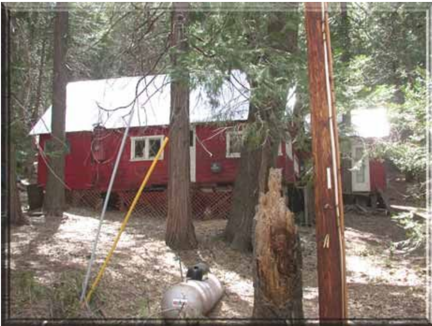
Figure 19: The entire home is built above the surface of the ground. Blowing embers will land under the house traveling through the lattice and openings seen under and to the left of the window. Photograph by Timothy Walsh
