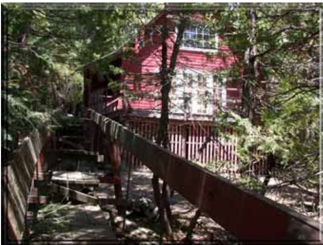
Figure 43: The rickety plank boardwalk up to 10812 Elm was very unstable and could become worse during a wildfire. Photo by Timothy Walsh.
