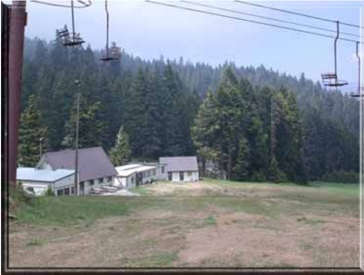
Figure 58: The commercial buildings that make up the Shirley Meadows Ski Area with excellent defensible space. Behind the building is pavement that is used as a parking lot during the ski season.
