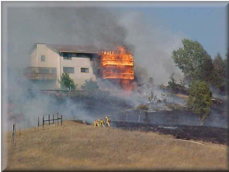
Figure 28: A fast moving grass fire ignited flammable ornamental vegetation under the first deck. It quickly spread to the deck above and throughout the house.
