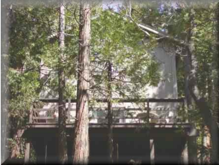
Figure 21: A typical home found in Alta Sierra; an open wood deck, wood siding, and fuel growing in close proximity to the house.
