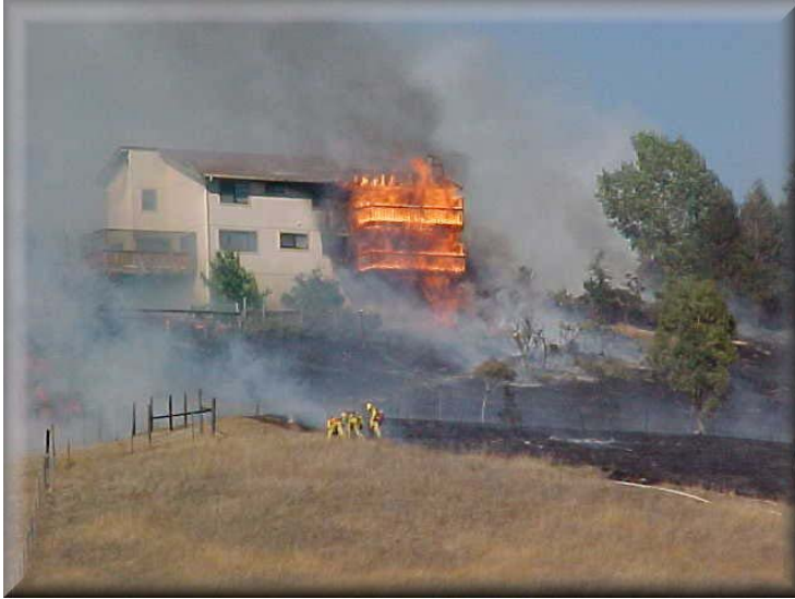
Figure 28: A fast moving grass fire ignited flammable ornamental vegetation under the first deck. It quickly spread to the deck above and throughout the house.
