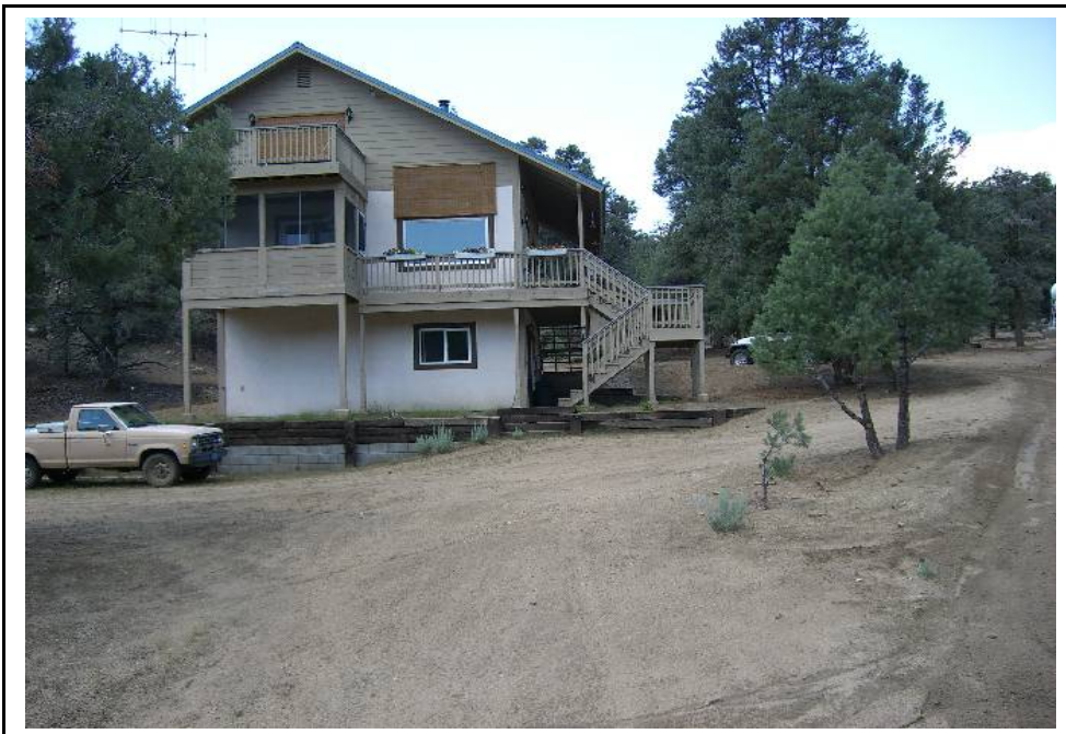
Structure pictured has good clearance, non-flammable siding, metal roof, composite deck, and emergency water supply with hydrant.
