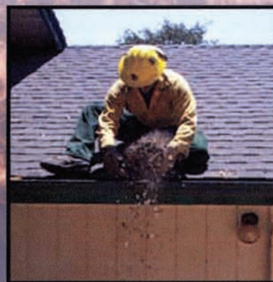
Clean out rain gutters and drainage pipes
